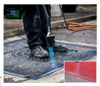
Designed for the application to asphalt roads to prevent water ingress and progressive fretting.
