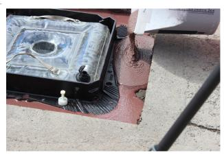
The inflatable device that acts as a dam allowing a flowable mortar installation around an access frame within seconds.
