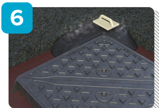
6 To provide longevity of service life in high stress areas such as braking and turning areas, use Enviro Mastic® Hot Applied Polymer Modified Mastic Asphalt.
