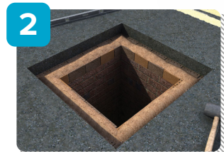
2 Old bedding mortar, loose bricks and debris are removed.
